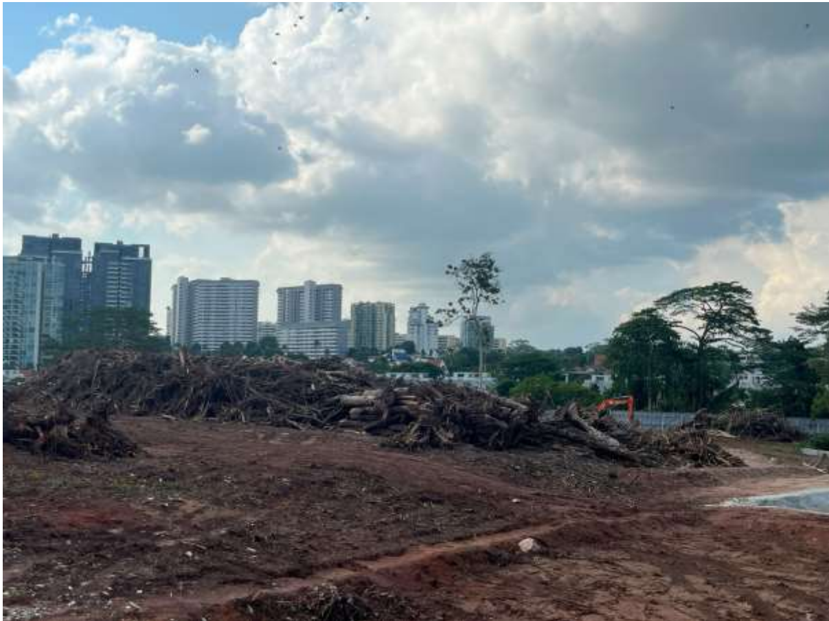
Image 3: Abandoned rubber plantation cleared for a block of flats (photo by author)
